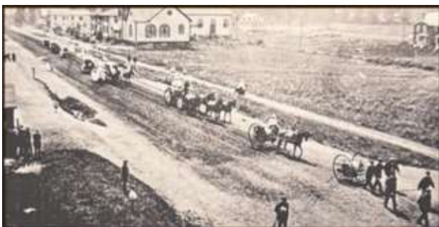
Construction of Delaware Avenue.
